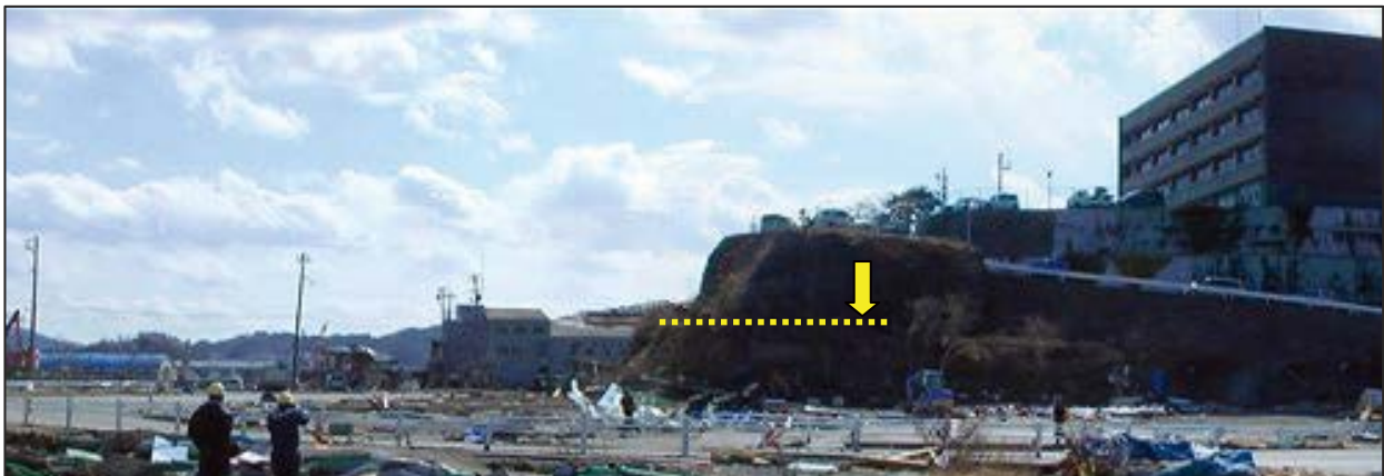
Photo 102 Traces of Tsunami (at point 102 in Fig. 3.2.83). Found drifts.
