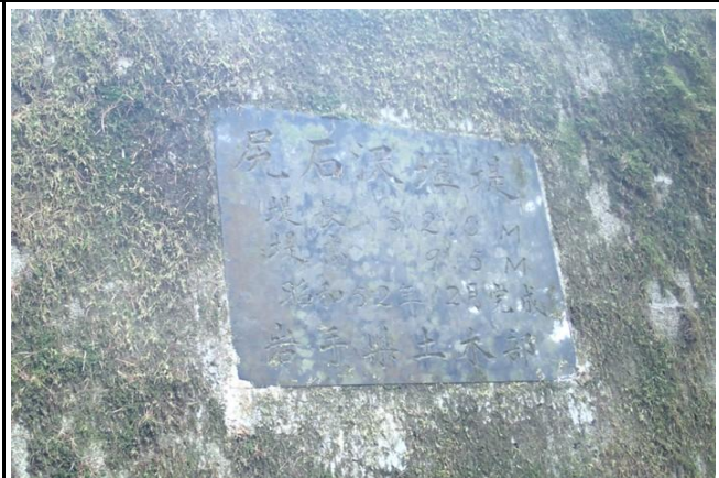
堰堤銘板(尻石沢堰堤, 堤長52m, 堤高9.5m, S52.12)
