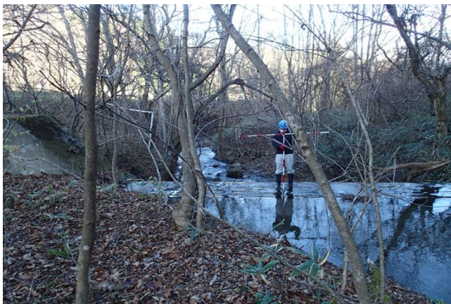
治山施設水通し(天端幅1.5m)
